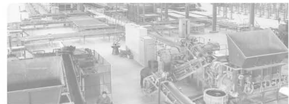
Workshops and production Lines
