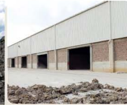
The semi-product indoor repository with storage capacity of 150,000 tons
